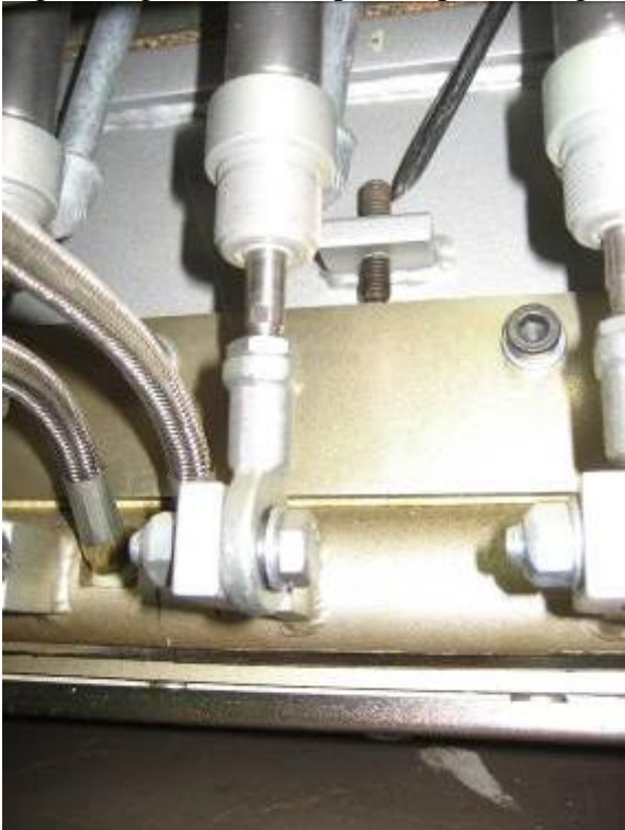
Tightening of Teflon rope/damper sealing
